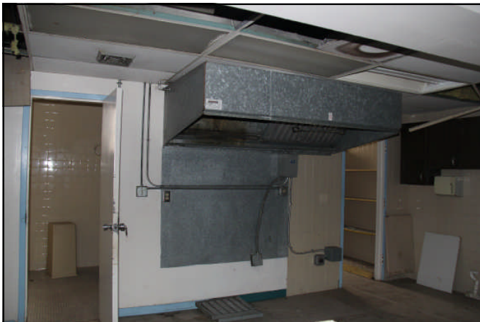
Former Kitchen Area
