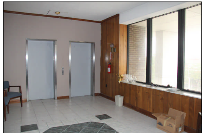
Upper Floor elevators
